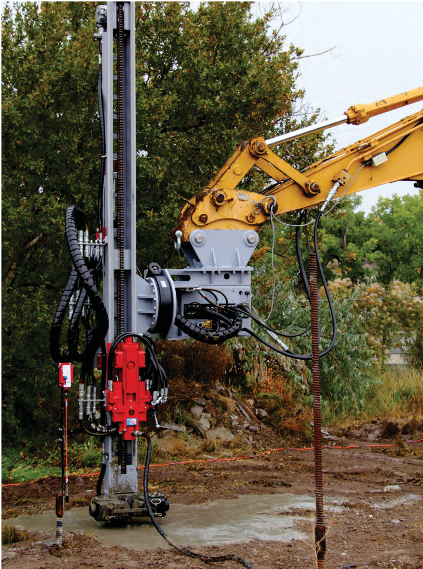
TEI DRIFTERS INCORPORATE A BUILT-IN SWIVEL THAT PUMPS THE GROUT DIRECTLY INTO THE POPULAR HOLLOW BAR SYSTEM
