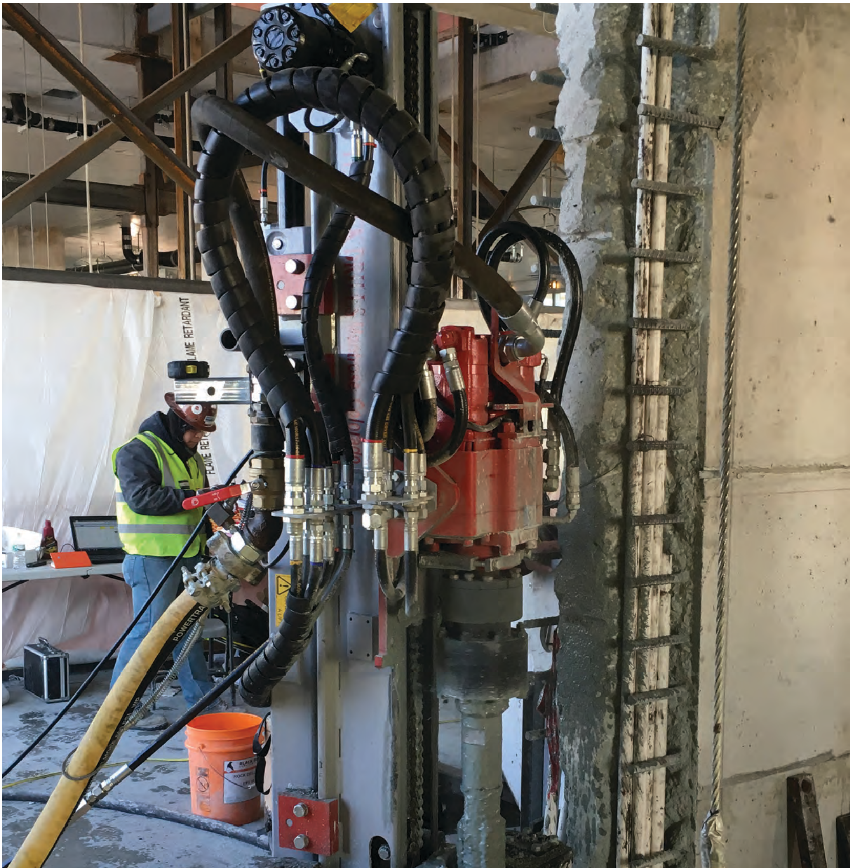
PD550 PORTABLE DRILL INSTALLING MICROPILES IN A HIGH RISE, BETWEEN FLOORS
