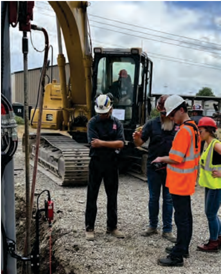
HOLLOW BAR INSTALLATION SCHOOL
