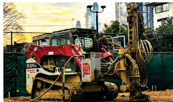
TEI SKID STEER DRILL ATTACHMENT
