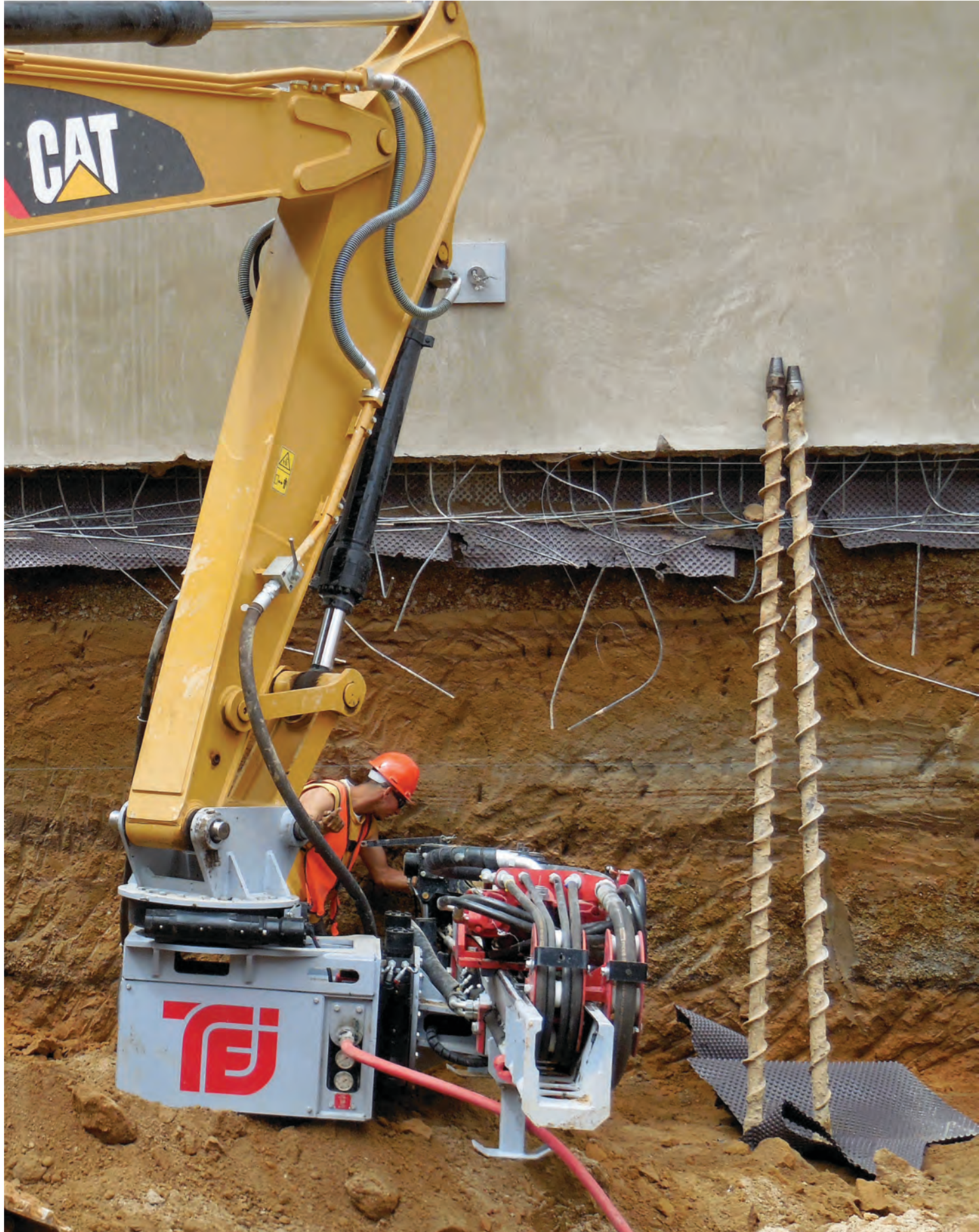
TEI EXCAVATOR ATTACHMENT IN USE FOR SOIL NAILING PROJECT
